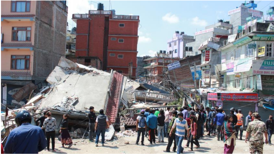
A scene from the aftermath of the 2015 Nepal earthquake. Rajan Journalist/Wikimedia Commons
