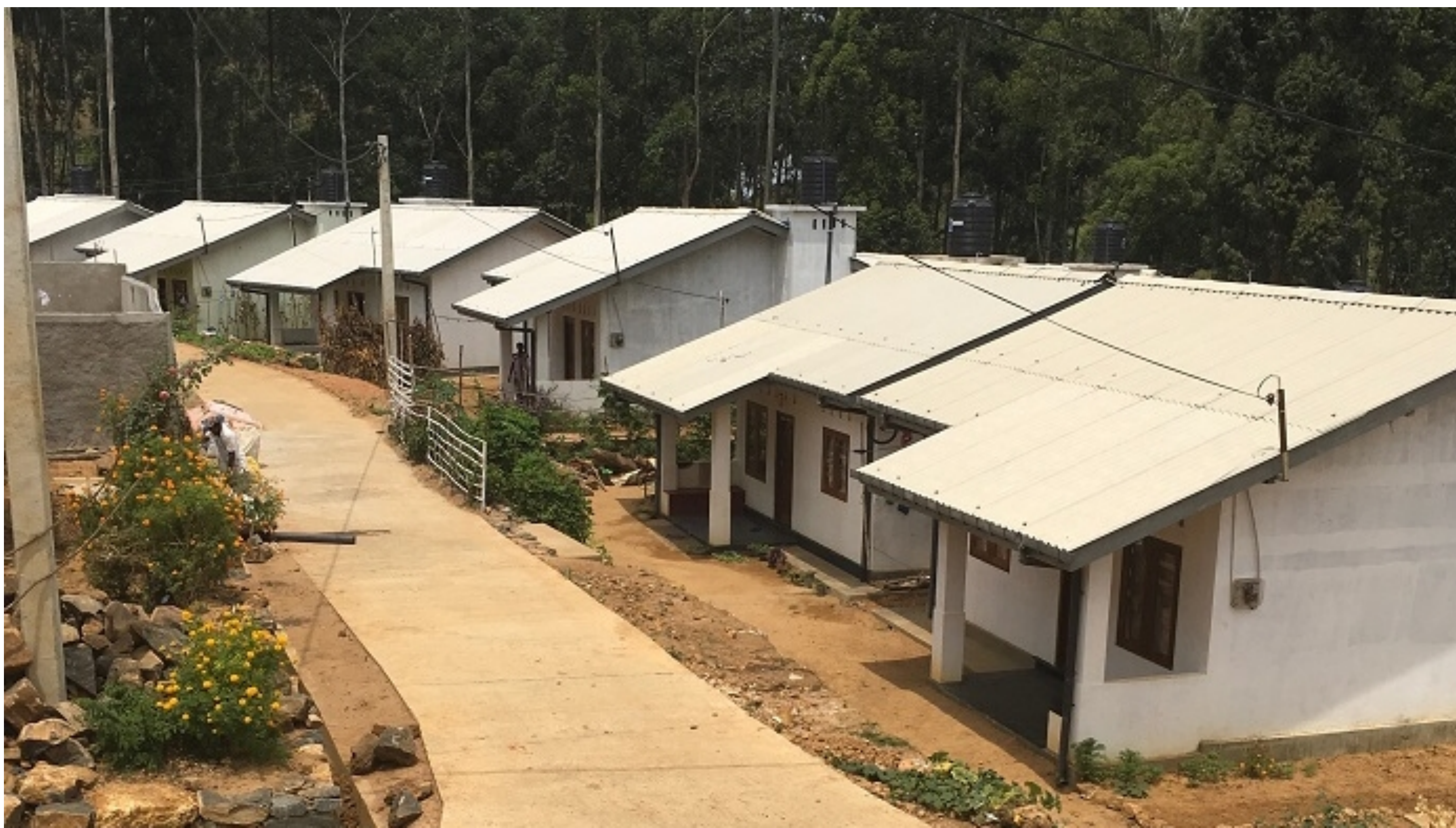
Relocation scheme of displaced communities due to Meeriyabedda landslide, Sri Lanka © Prof. Dilanthi Amaratunga
